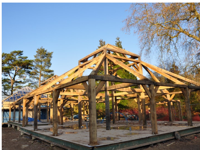
The green oak frames were constructed in Devon and erected onsite.
