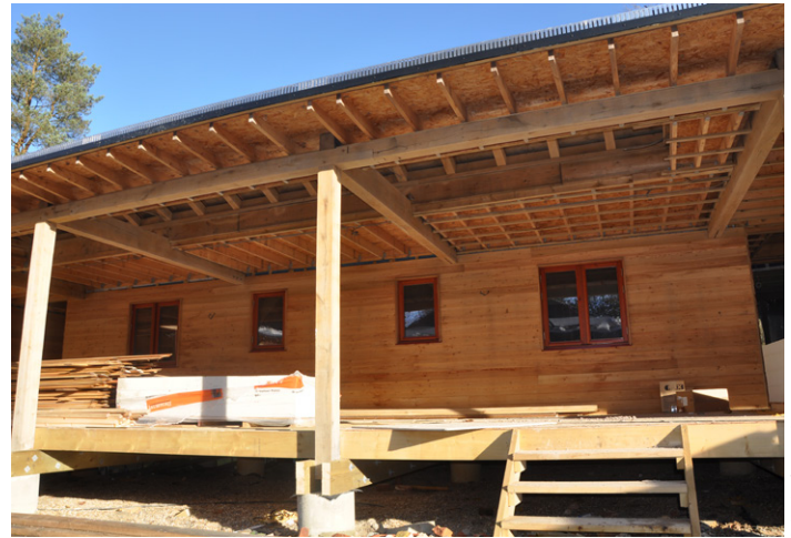
The flat roof over the veranda will be covered with sedum
